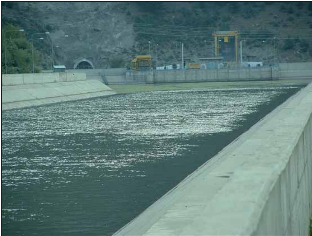
10. Canal Leading to Headrace Tunnel
