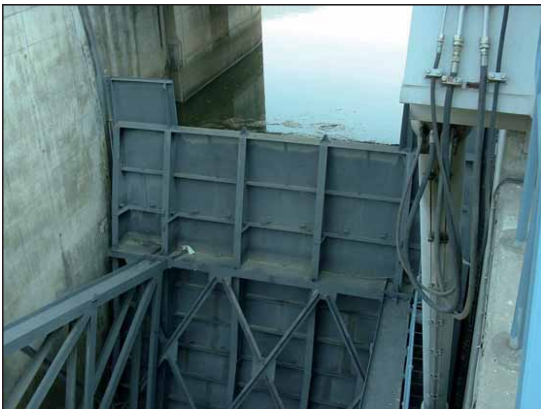
5. Radial Gate at Uri Barrage
