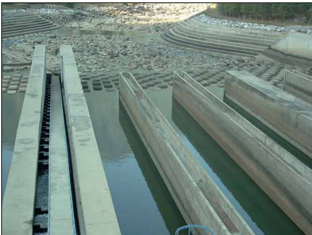
14. Fish Pass (left of picture) at Uri Barrage
