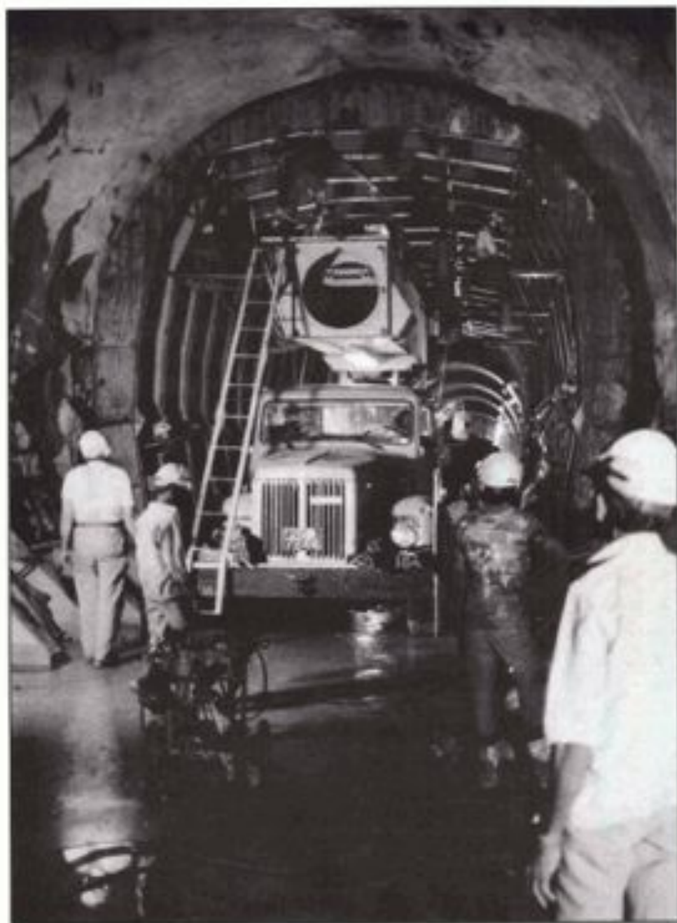
Concrete lining of a tunnel. Considerable costs could have been saved by using unlined low-pressure waterways. Photo: Skanska, Björn Enström
