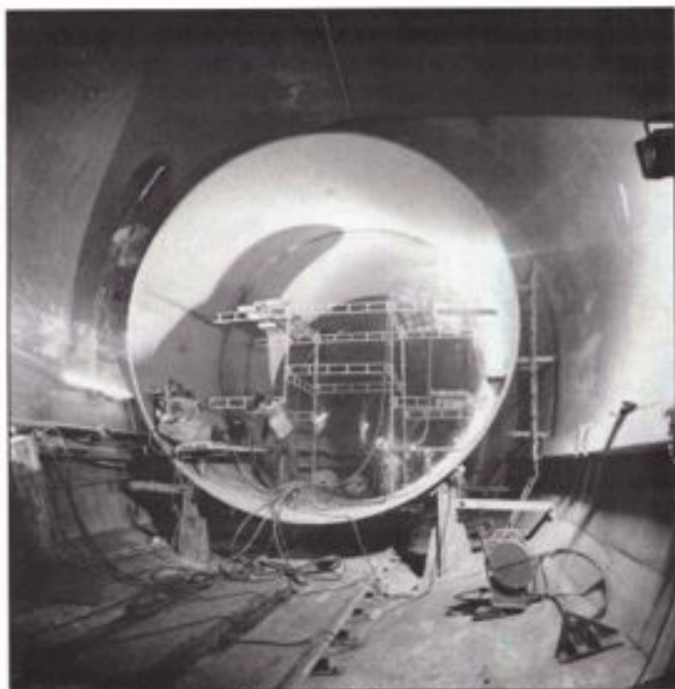
Steel lining of the pressure shaft, Kotmale 19866. Photo: Skanska, Björn Enström Shortly after the first filling of the waterways there was an excessive leakage from the pressure shaft into the powerhouse area. In the period from March 1985 to May 1986 the power plant was operating intermittently. The plant was then closed for 18 months to steel-line the entire pressure shaft and the inclined tunnel. Without delays or repair costs Kotmale would have had a considerably higher economic return. See table 11.9
