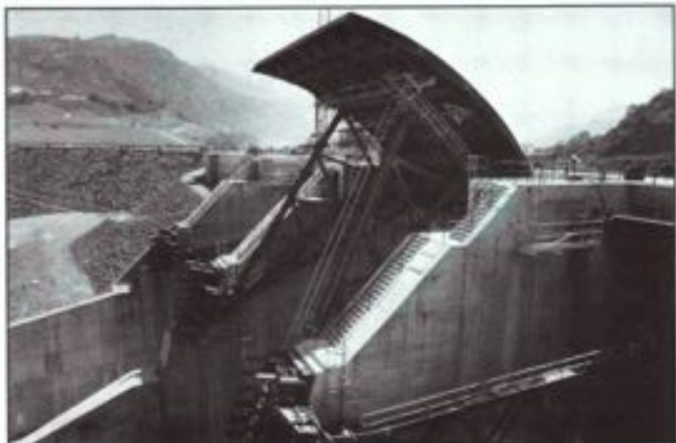
The three flood-gates are convex in shape to better withstand the pressure from the water masses. Beneath them lies the spillway that leads the water back to the river channel. Photo: Jan E Carlsson, SIDA Photo Archives
