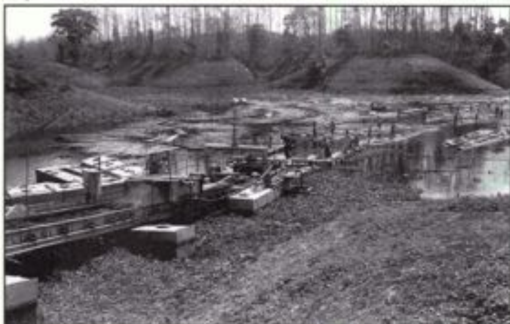
The chipping station at Kaptai is functioning well, but used only at half capacity due to shortage of timber. Photo by Karlis Goppers/SIDA Photo Archives.
