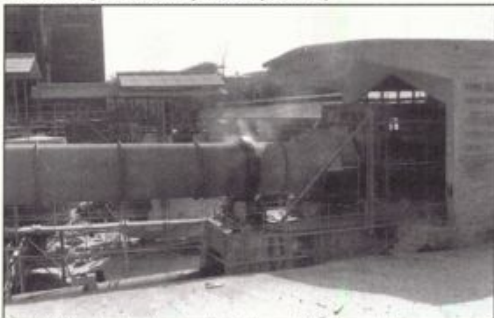
Inside KPM pulp plant. Photo by Karlis Goppers/SIDA Photo Archives.
