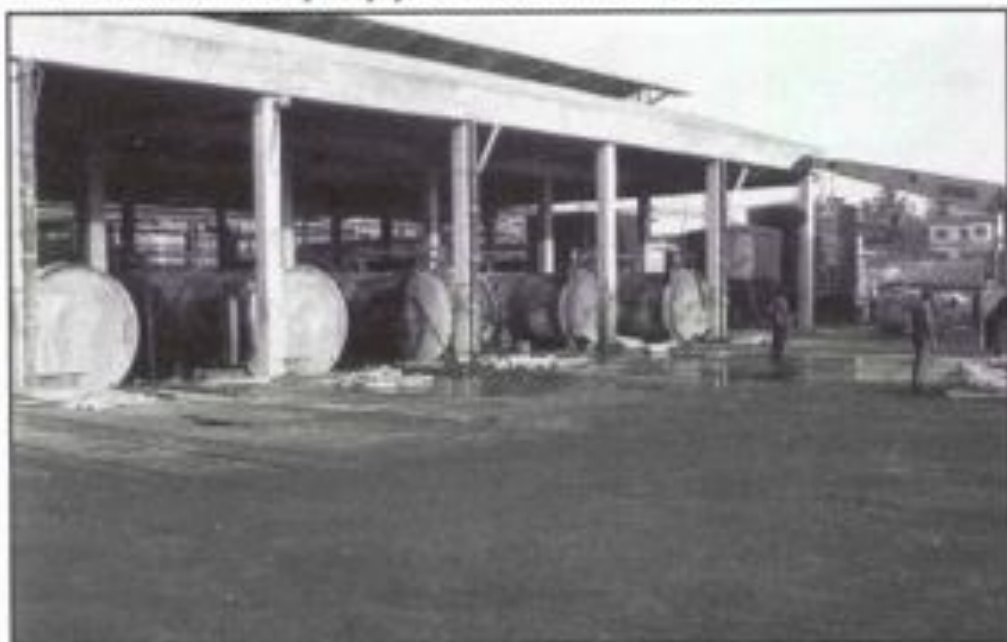
Khalna Newsprint Mill: Renovation of boilers was part of the rehabilitation program. Photo by Karlis Goppers/SIDA Photo Archives.
